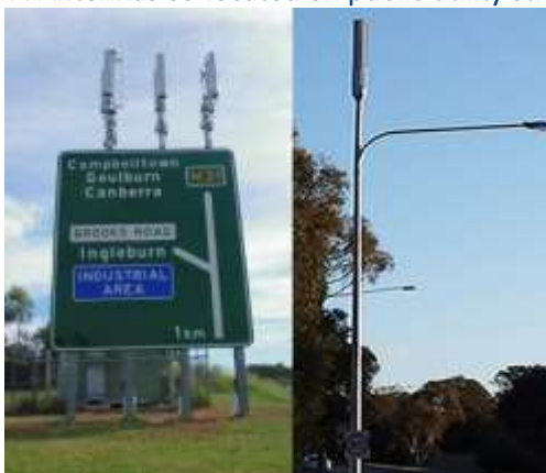
Figure 7: Antennas co-located on public utility structures
