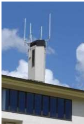
Figure 4: Omnidirectional antennas on a rooftop
