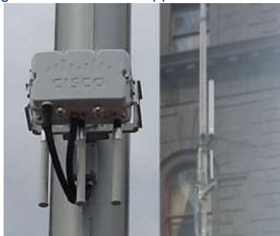
Figure 5: Wi-Fi transmitter (L) small cell antenna (R)
