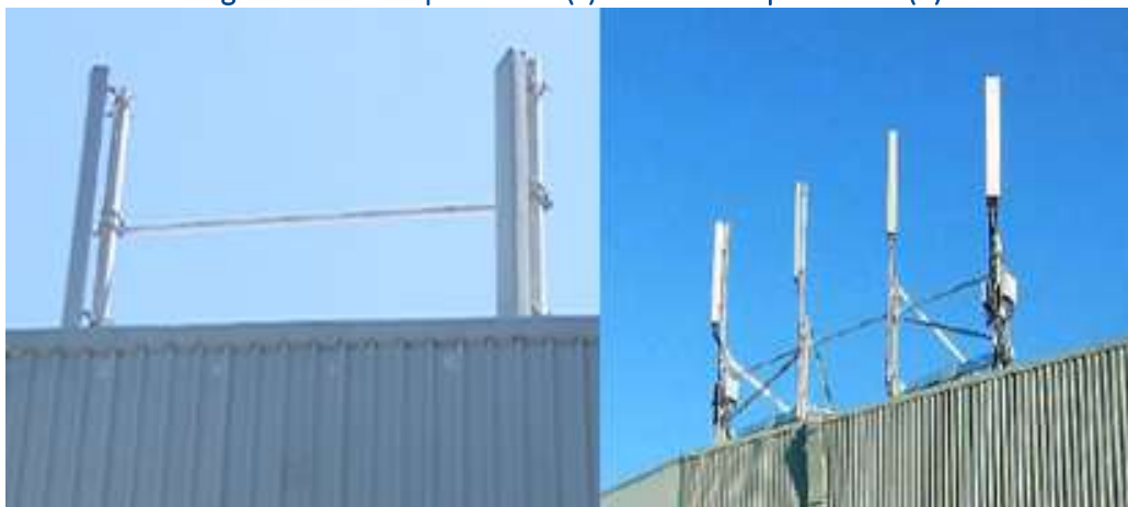
Figure 3: 3 metre protrusion (L) and 5 metre protrusion (R)
